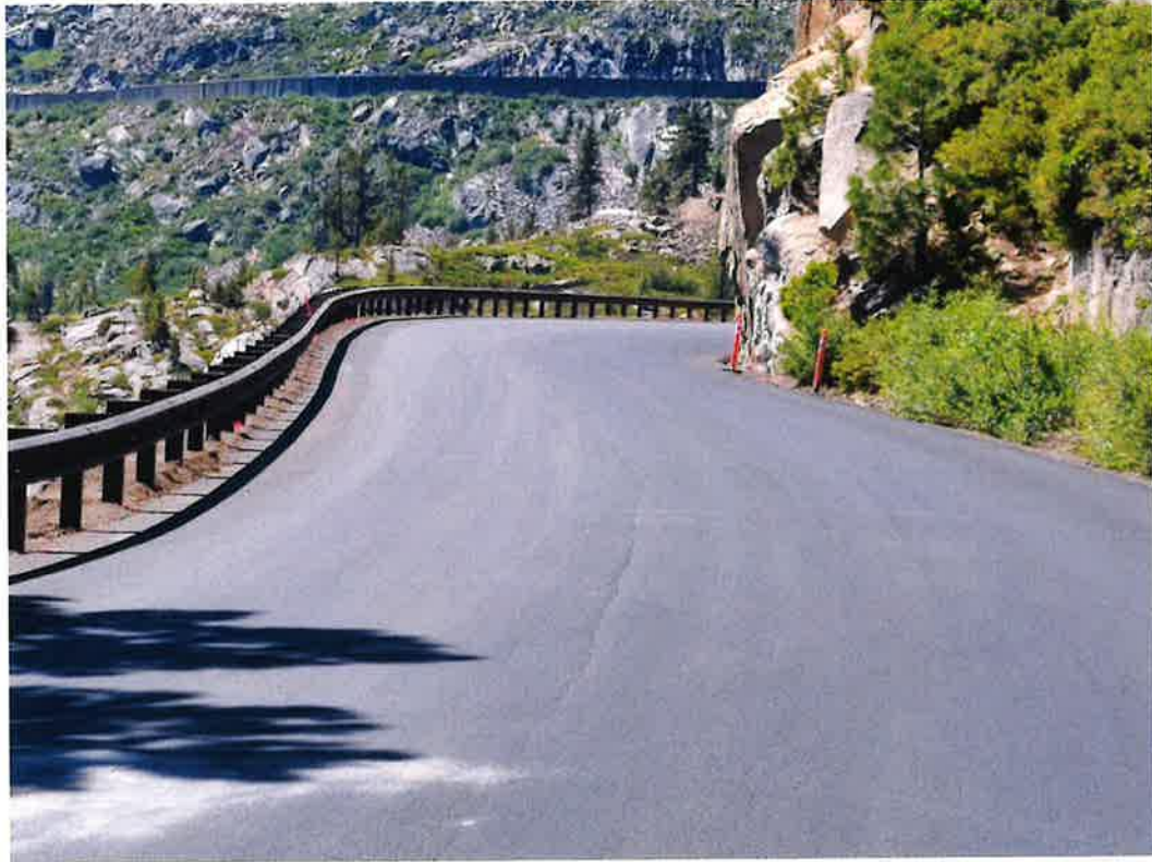
Widening Donner Pass Road
